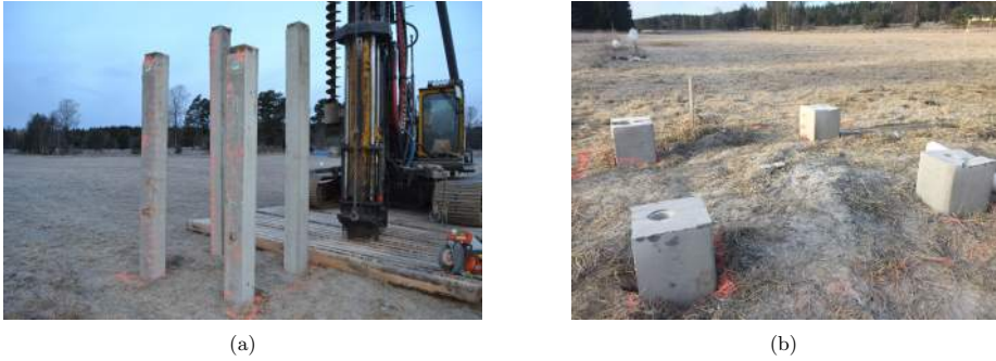
Figure 3: Impact driven concrete piles installed at the site (a) in full length before cutting illustrating the difference in driving depth between the piles and (b) when levelled.
